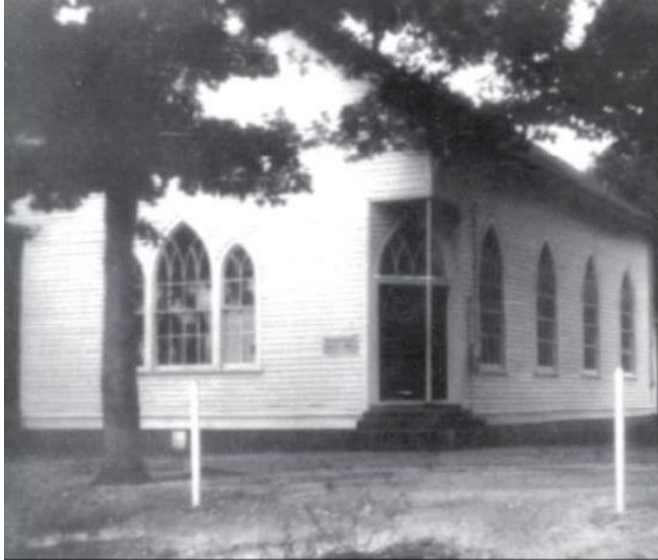
An undated photo of the church shows the diagonal entrance. The arched side windows remain today.
