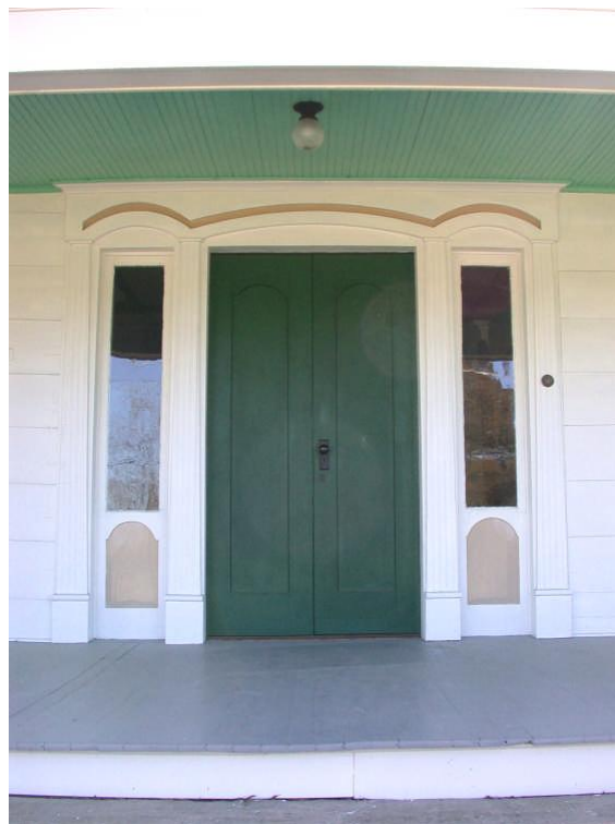
Front entrance detail
